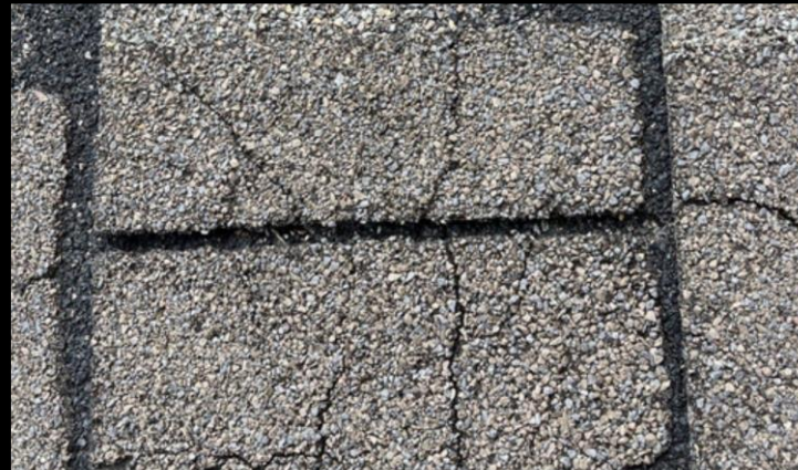
Cracking or Splitting
