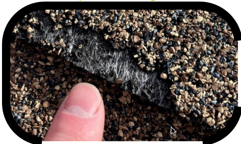
Exposed Fiberglass
